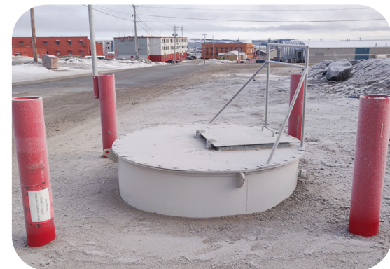
Installed steel manhole
