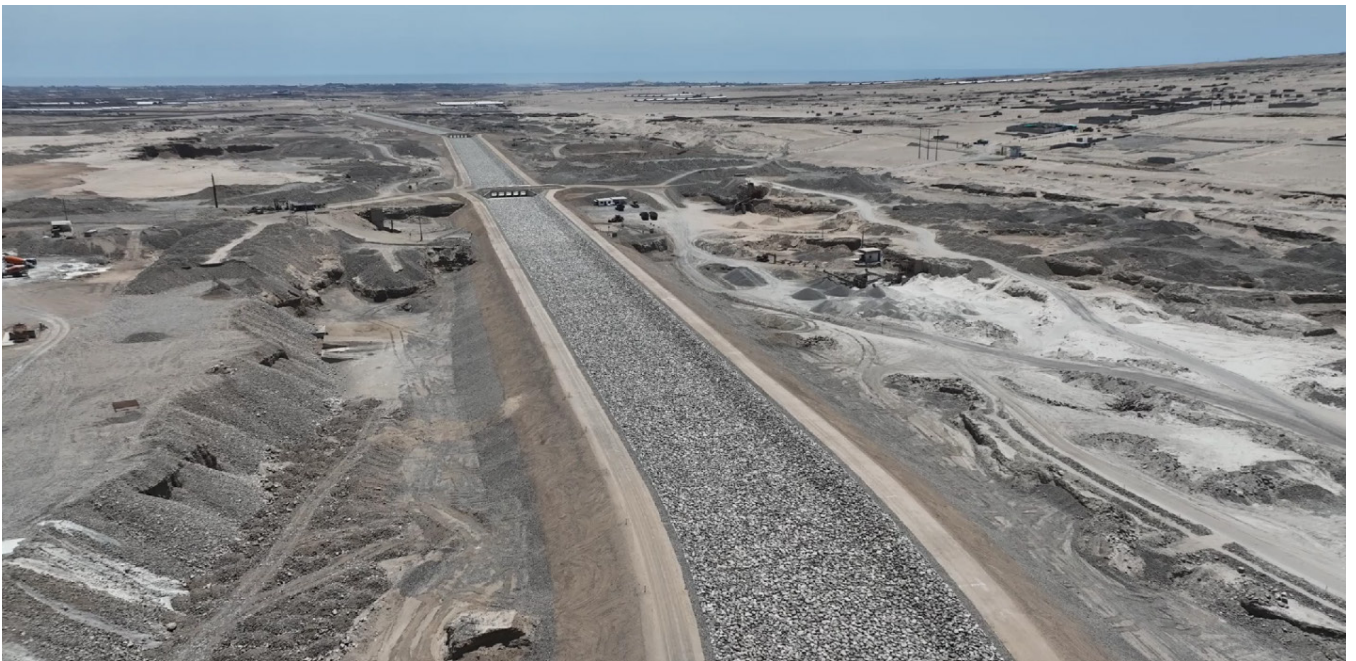
Canal crossing quarries in operation
