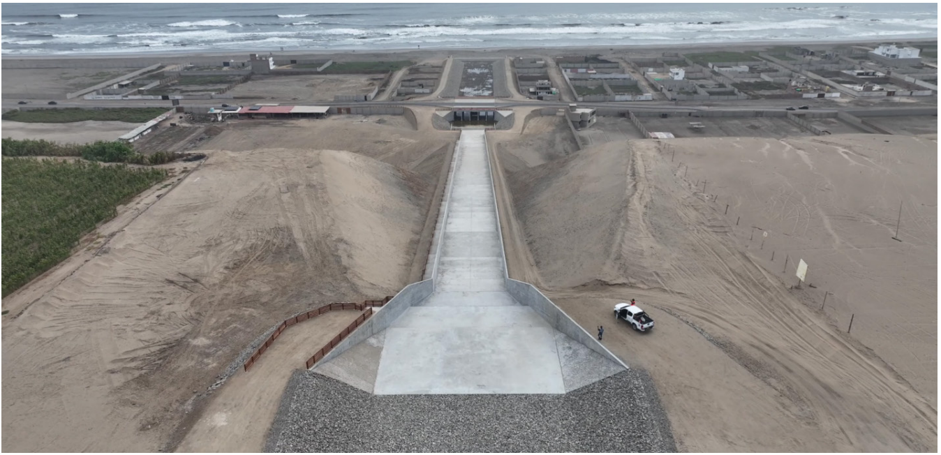
View of the discharge structures at the seacoast
