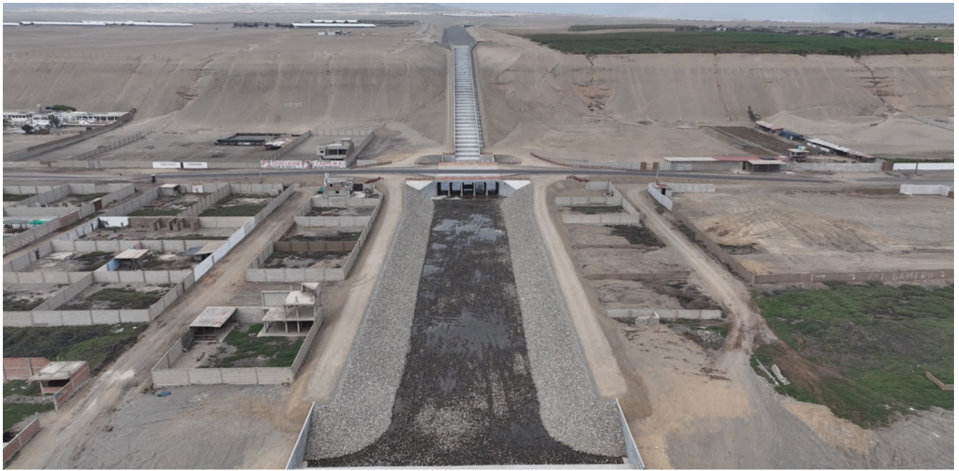
Downstream view of the discharge structures, photo taken from the beach
