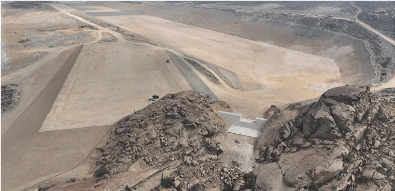
View of the headworks from downstream of the spillway
