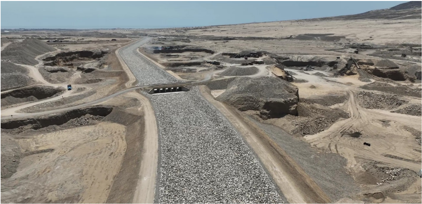
Canal crossing quarries in operation
