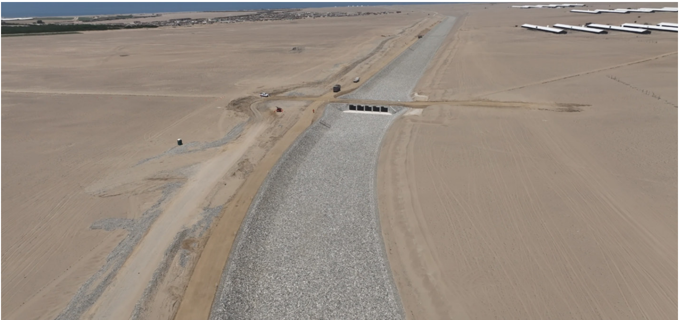
Downstream section of the canal, before junction with the discharge structures
