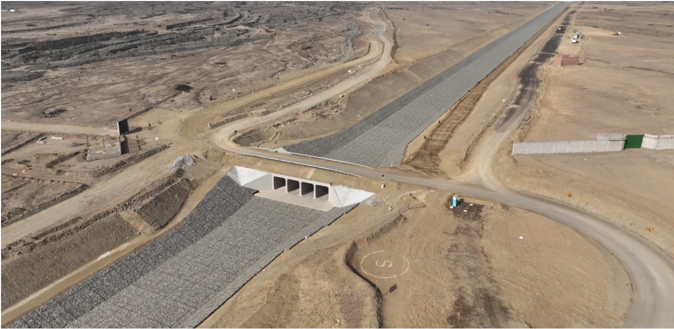
Downstream view of a concrete culvert for road crossing the canal
