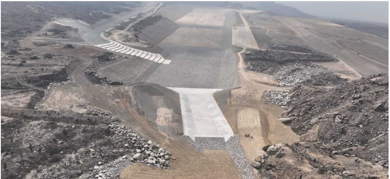
View of the headworks
