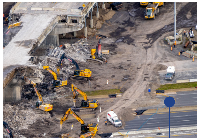
Above: mechanically deconstructing the spans, girders and piers piece by piece. Below: Some of the more than 4,000 salvaged rivets.
