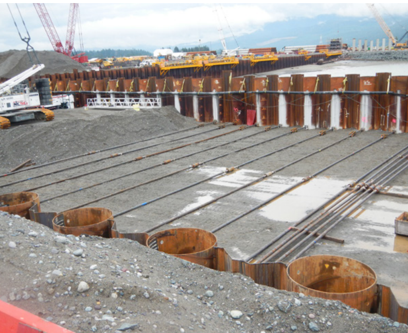
■ Installation of tie-rods on MOF West wall
