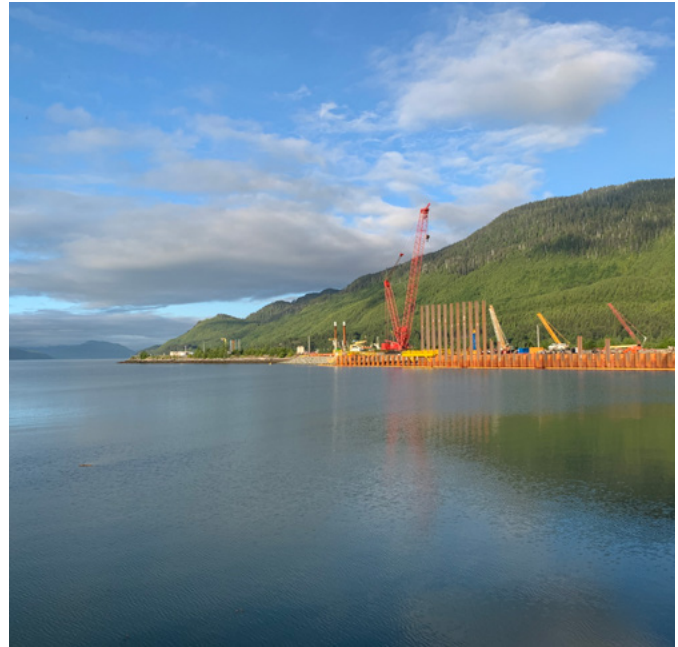
■ West bulkhead wall of MOF during construction
