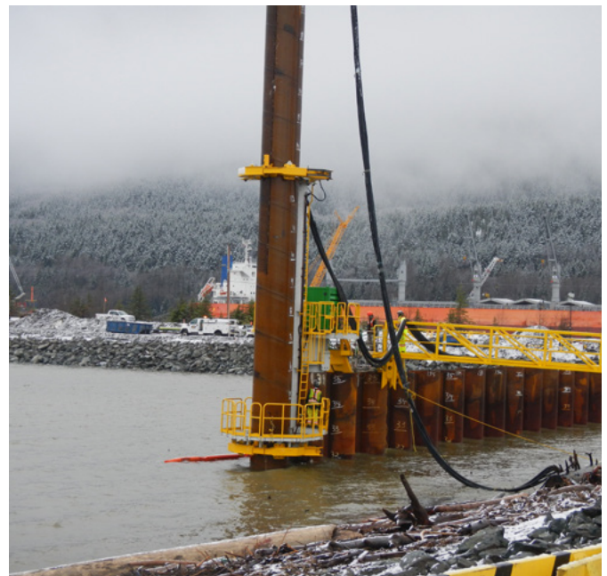
■ Installation of first pipe piles on North wall
