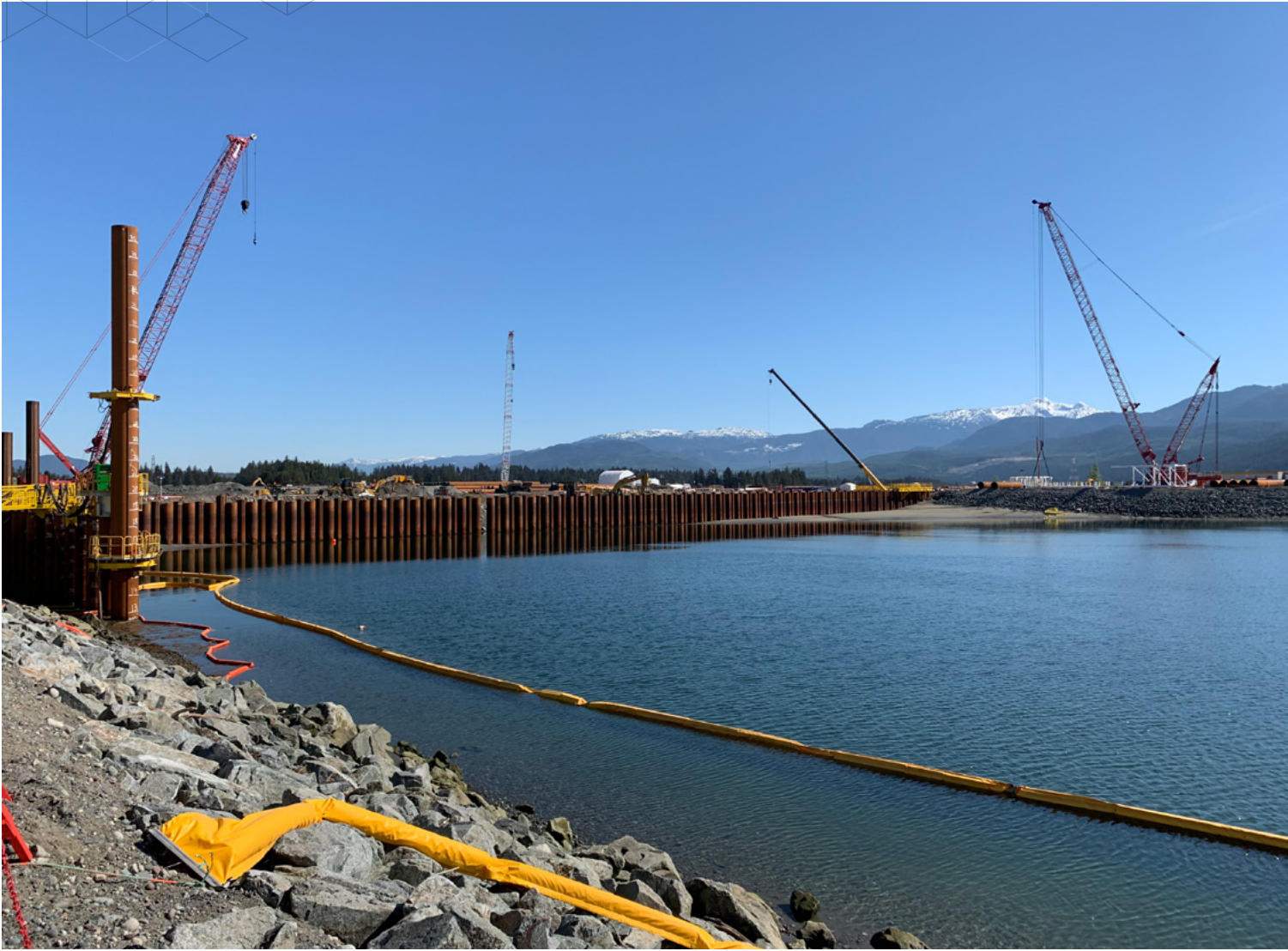
■ North bulkhead construction of MOF before dredging
