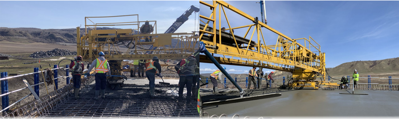
Concrete Deck Construction on Cache Creek Bridge
