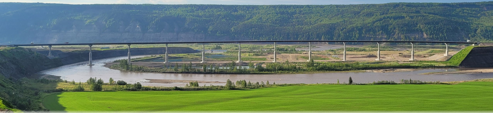
Completed Halfway River Bridge
