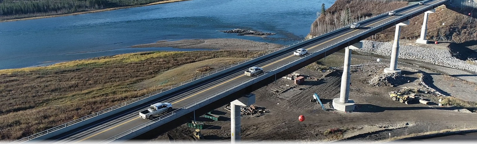
Farrell Creek Bridge Opening
