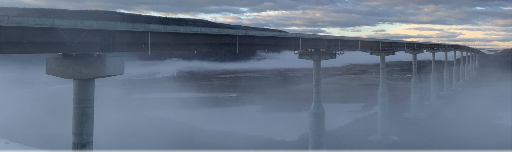
Completed Halfway River Bridge Rising Above the Morning Mist
