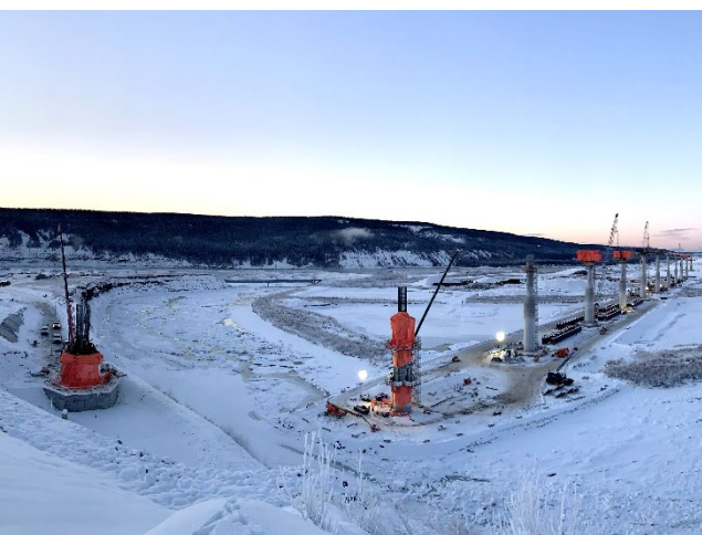
Pier Construction in Harsh Northern Climate
