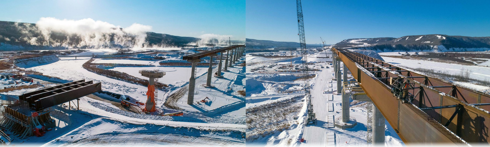
Construction of the Halfway River Bridge in Cold Northern Climate
