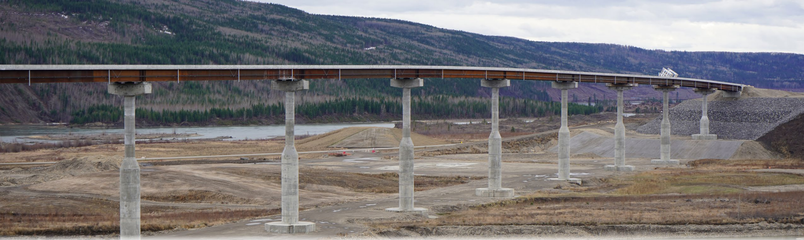
Tall Piers of the Halfway River Bridge before Site C Reservoir Filling
