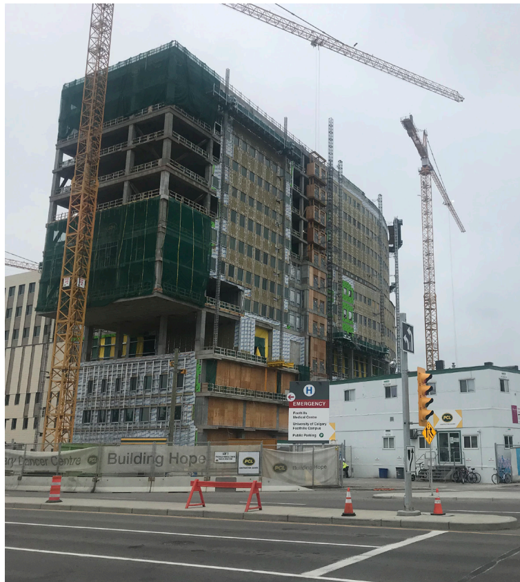
▲ Cantilevered Floor Plates
